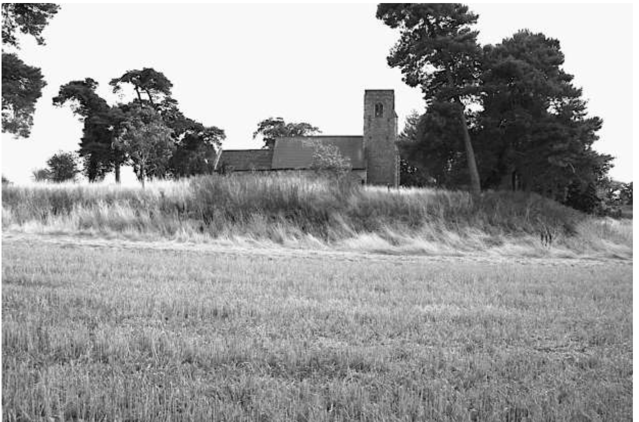
Saint Lawrence Church on its levelled site overlooking Stone Street
